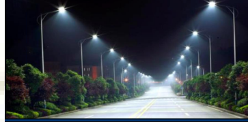
LED Street Lighting with < 30m pole spacing
